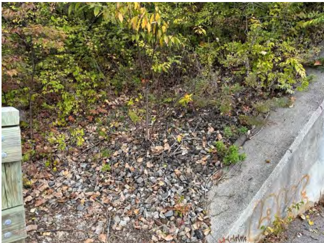
AOI B, Riprap along hillslope. Lat. 39.98121, Long. -82.95254
